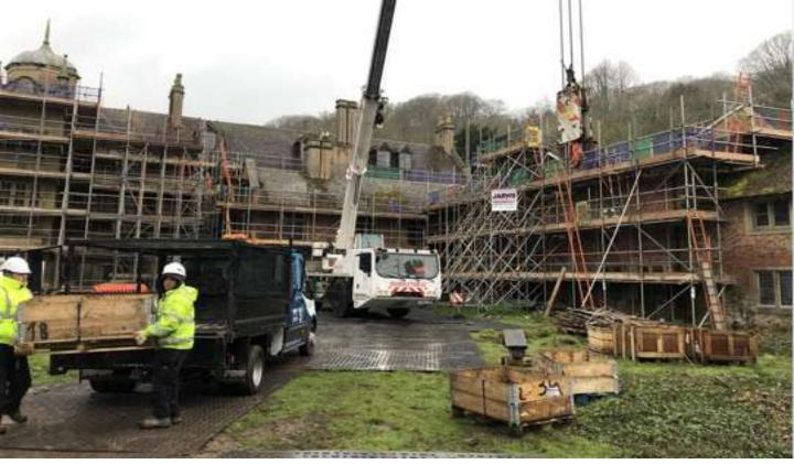
The project began slowly in late 2018 with initial site surveys and enabling works to make the property safe to enter. This included extensive removal of accumulated rubbish and debris, temporary repairs to provide safe illuminated walkways and work areas. Full external scaffolding was installed to permit inspection of the property and to reinforce the collapsed wing to aid debris clearance.
